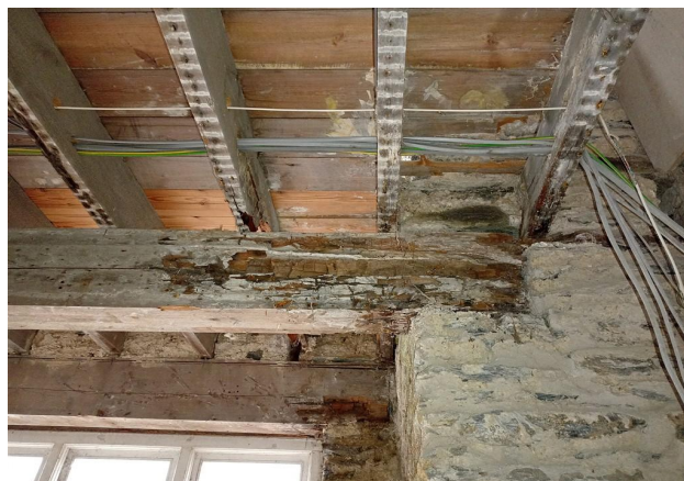
Two Rotten Structural Beams
