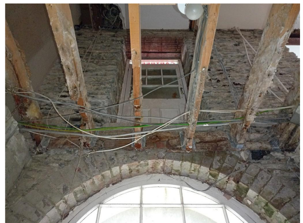
Rotten Joists On 1st Floor
